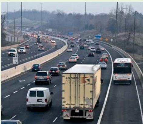
Bus Bypass Shoulders can allow for fast and reliable transit service on busy highways.
